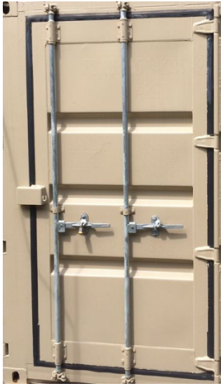
Figure 31. Sample door with gaskets protecting against EMP threats
